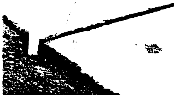
Fig. 3.2.2.1 — Faulting (stepping)
